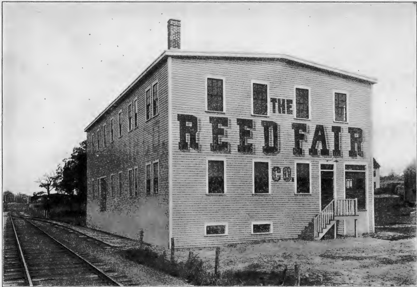
The New Building of the Reed Fair Co. on Rose St., Salem, Mass.
